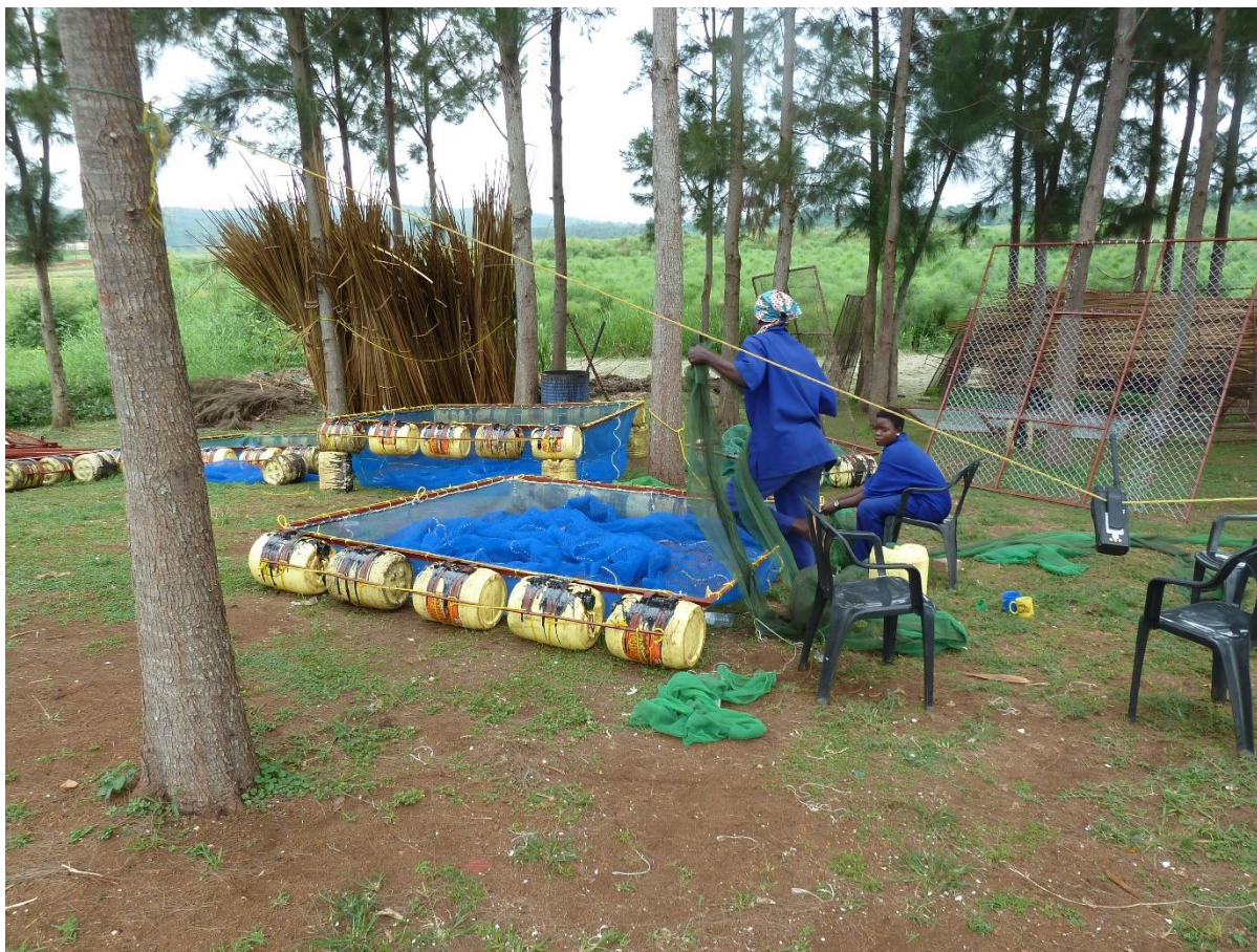
Figure 11: Attaching nets to simple metal frame cages
